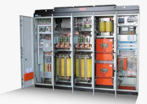
The racks include power and water distribution to the power supplies, a general and individual circuit breakers and a digital flowmeter with a water temperature measurement, interlocked with the power supplies. The power supplies feature an Ethernet interface, along with custom digital I/Os and remote voltage sense.
